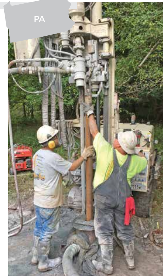
Connor Neely, driller (left), and Chris Chronister, field superintendent, add a drill rod during the 5-inch air percussion drilling.
