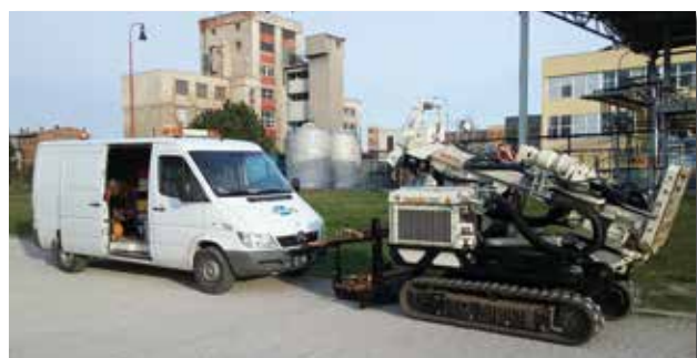
On site for the MIP investigation were Dekonta's MIP support vehicle; a 7822DT was used to advance the MIP probe and collect soil samples.
