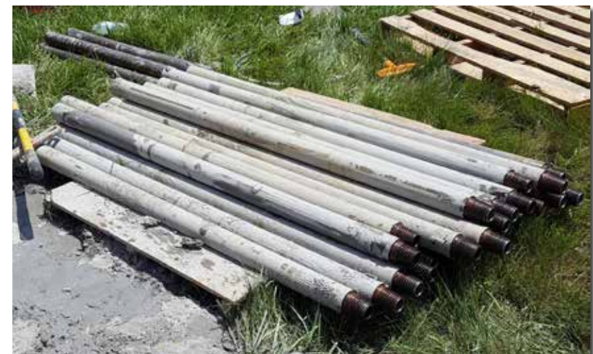
Five-foot drill stem sticks after removal using the Geoprobe® hydraulic breakout system.
