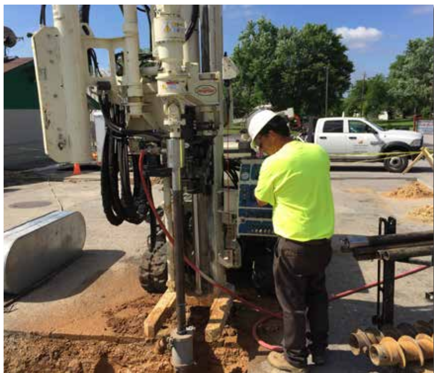
A GA4000 augerhead provides the power and rotation needed for air rotary drilling with the 7822DT.
