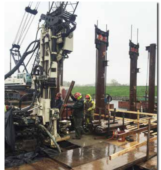
(l to r) Randy Crandell (at the controls), Shaun Biggs, and Chris Ruschmeyer add a stick of 6-in. casing to be advanced over a 4-in. core barrel using the 8140LC rotary sonic on a barge.
