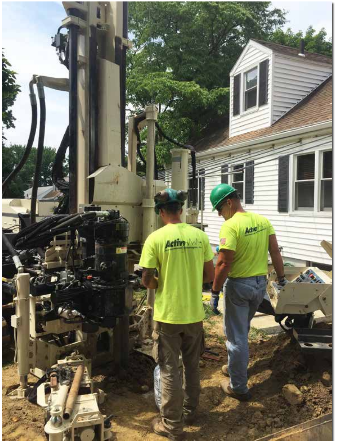
Nick Kolenda (left) and Tom Hartwell, Drillers for Active Environmental Technologies, use a 3230DT to install 2-inch monitoring wells in a residential area. Monitoring wells were installed to determine potential groundwater impact.
