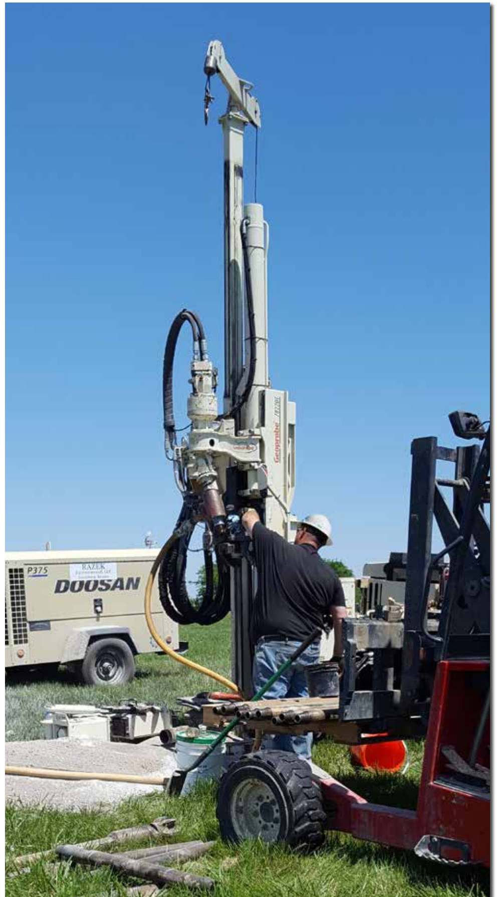
Tony Poulter, Vice President and Co-Owner of RAZEK Environmental, installs geothermal loops in 6-in. diameter, 150-ft. deep bores with a 7822DT. Tripping out of the boring in 5-ft. increments "worked flawlessly."
