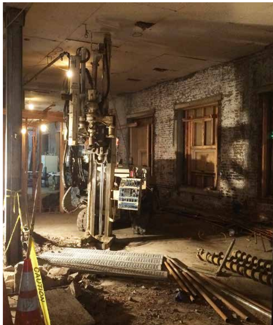
(above and right) Very little head room. The vertical work space for this 7822DT was only 13 feet, but it was enough for Hynes & Associates to collect foundation information for structural modifications for the building.
