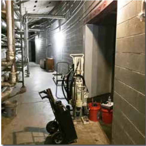
GeoTest Services collected approximately 30-in. long concrete cores with a 420M as part of the project for five limited access borings at the University of Houston inside the main auditorium of the Hofheinz Pavilion. The concrete coring was through hard rock aggregate concrete found in the older structures in Houston.
