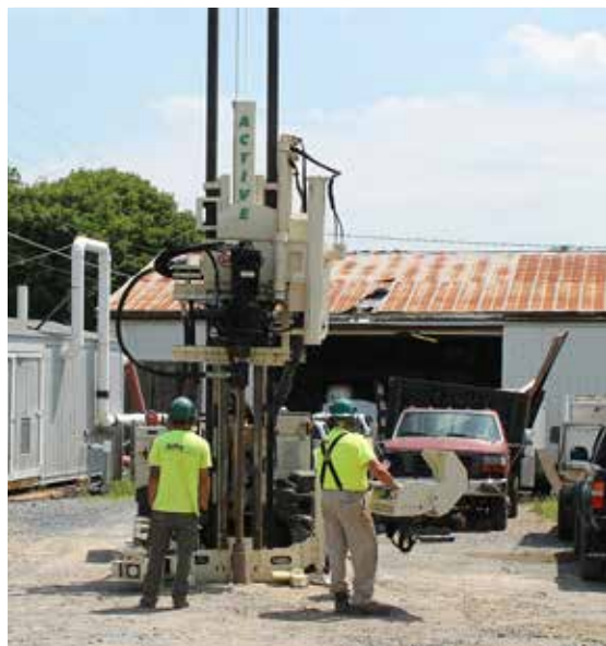
Nick Kolenda (left) and Tom Hartwell, Drillers for Active Environmental Technologies, use a 3230DT to install 2-inch monitoring wells in a residential area. Monitoring wells were installed to determine potential groundwater impact.
