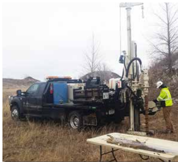
(right) Midwestern Drilling's 7822DT is lifted over a pile of rubble caused by a train derailment. (above) Dusty Schroeder, President of Midwestern Drilling in Holloway, MN, installs monitoring wells with a 7800 at a local landfill.
