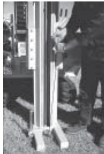
Once the E-log is completed, the signal cable is snapped off of the expendable SC310 probe before the Grout Pull Cap (GS1254) is attached to the rod string.
