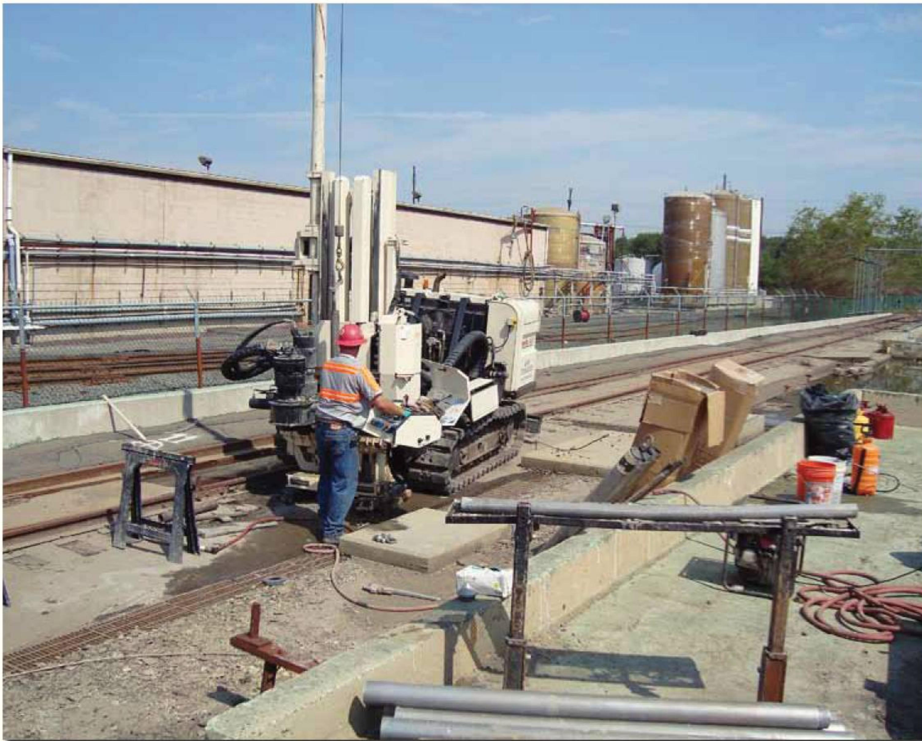
Chris Lacko, Field Operations Manager for ARS Technologies in New Brunswick, NJ, uses their 8040DT at an abandoned manufacturing facility, continuous coring with DT325 tooling to over 100 feet.
