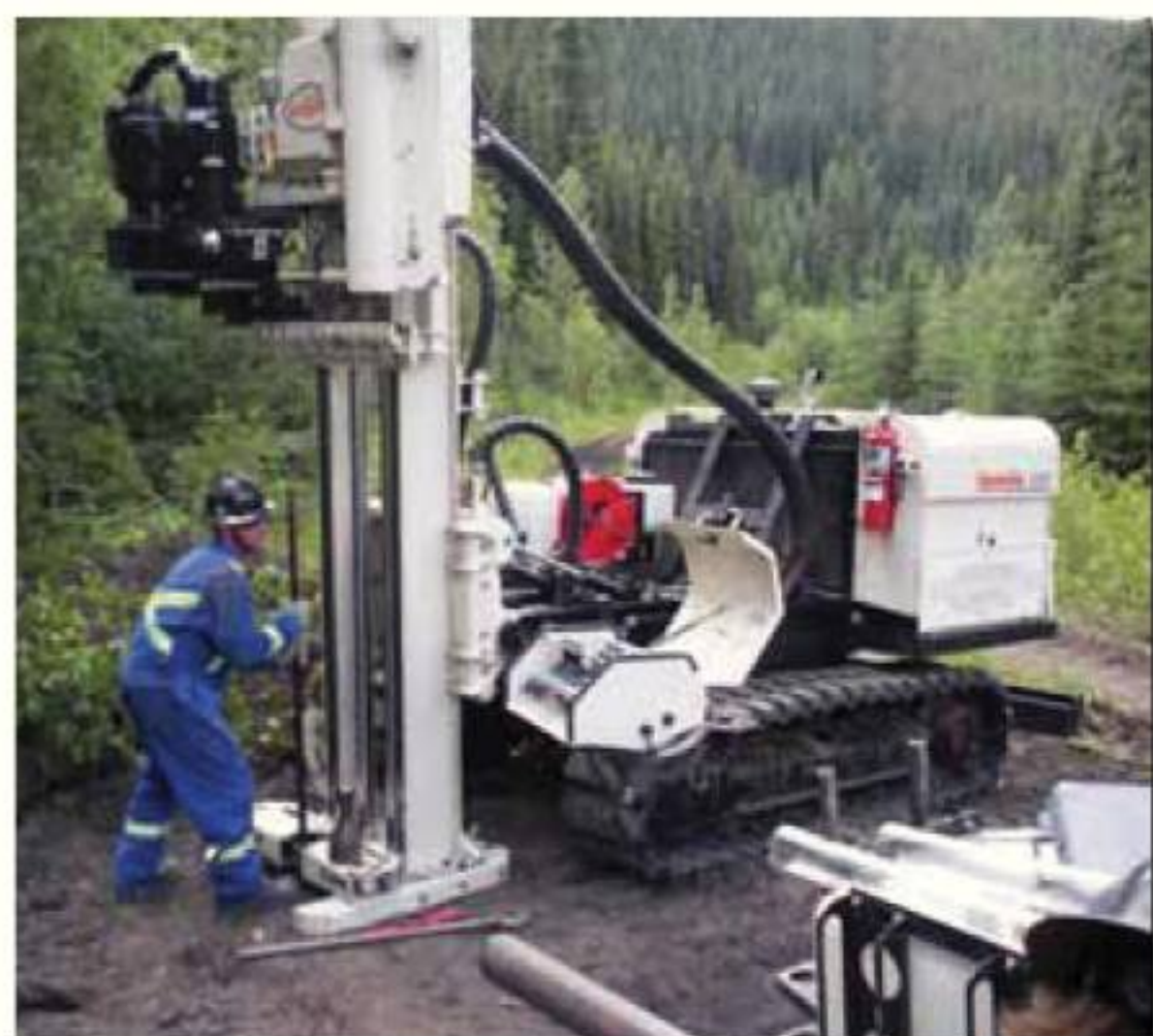
Chris Lacko, Field Operations Manager for ARS Technologies in New Brunswick, NJ, uses their 8040DT at an abandoned manufacturing facility, continuous coring with DT325 tooling to over 100 feet.
