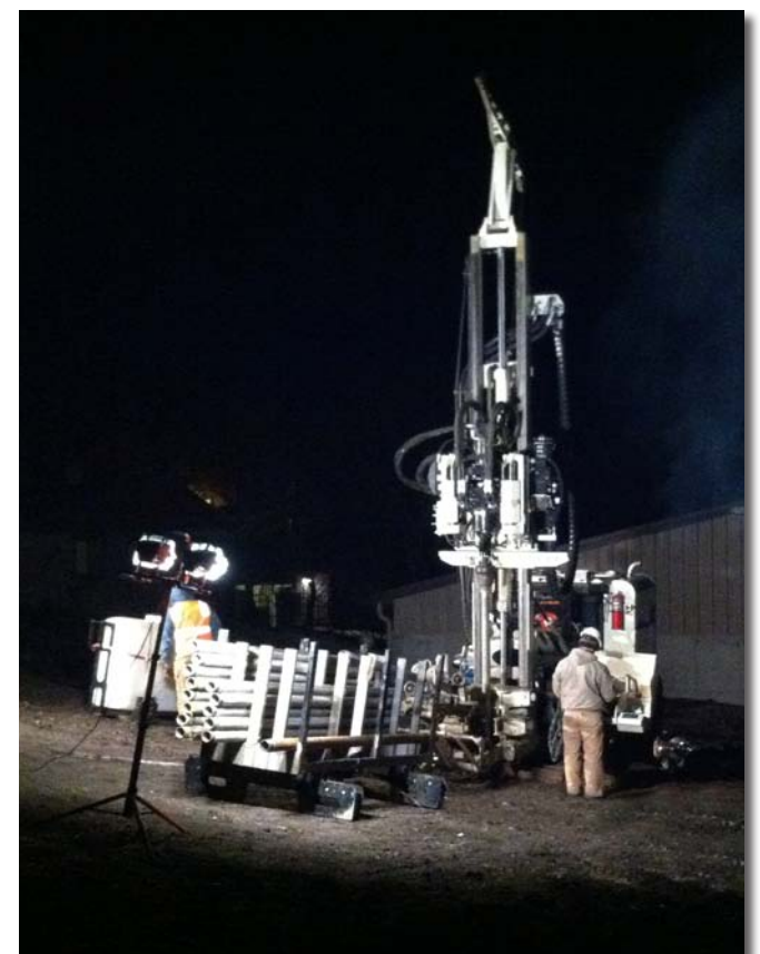
No, it's not a lunar landing! Team Geoprobe works at the geothermal loop installation site in the really cold, early morning hours.
