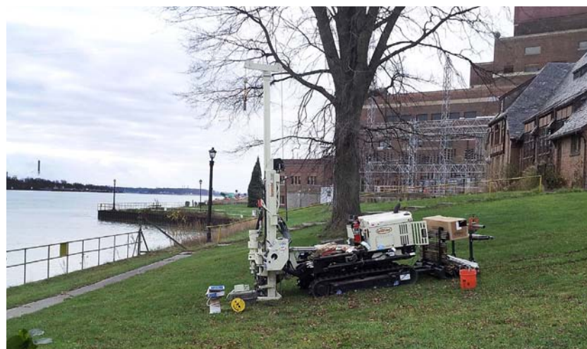
The Stearns Drilling 7822DT, with Tom Ulrich the one-man drilling crew and photographer, works in Marysville, in southeastern Michigan, at a Detroit Edison coal plant, built in the 1920s. Tom was collecting soil samples and setting 1.0 in. PVC temporary monitoring wells. Marysville is on the western shore of the St. Clair River across from Corunna, Ontario in Canada.
