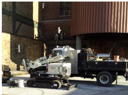
The Stearns Drilling 7822DT, with Tom Ulrich the one-man drilling crew and photographer, works in Marysville, in southeastern Michigan, at a Detroit Edison coal plant, built in the 1920s. Tom was collecting soil samples and setting 1.0 in. PVC temporary monitoring wells. Marysville is on the western shore of the St. Clair River across from Corunna, Ontario in Canada.
