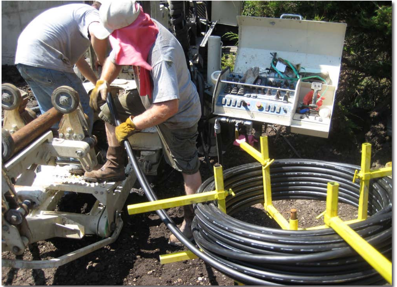
Using a Geoprobe® 8140LS Rotary Sonic, Jed Davis, Geoprobe® Tooling Engineer, prepares geothermal loop for installation at a new dining hall construction site. As things worked out, the field team made a single test hole in the hottest part of summer, then completed the other 14 holes in the grip of winter. Ah! The joys of drilling!
