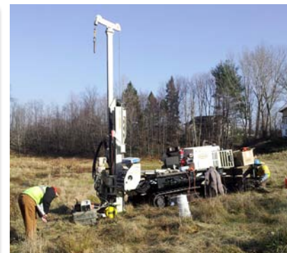
The Stearns Drilling 7822DT, with Tom Ulrich the one-man drilling crew and photographer, works in Marysville, in southeastern Michigan, at a Detroit Edison coal plant, built in the 1920s. Tom was collecting soil samples and setting 1.0 in. PVC temporary monitoring wells. Marysville is on the western shore of the St. Clair River across from Corunna, Ontario in Canada.
