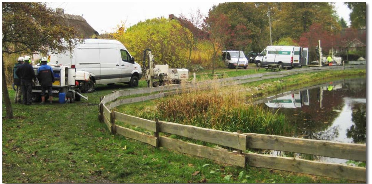
NIRAS set up two of their Geoprobe® 6610DT rigs in the community park for the MiHpt Investigation. The MIP wagon and probe unit are set up at the SK04 location. Note large glacial erratic boulders in the park. A machining/manufacturing facility located next to the park had used PCE in their machining and clean-up processes. The PCE was released to the environment, and the soil and groundwater in the area was contaminated.
