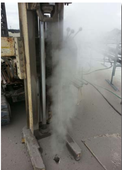
Adding to the already hot/humid ambient temps, 200 degree F steam is seen pouring out of a borehole after sampling tools were pulled.
