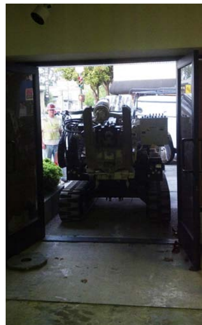
Glenn Reiss, Owner/Geologist with Vapor Tech Services in Hayward, CA, guides a 7822DT through a building entrance. Seventeen remediation wells were installed inside the building.
