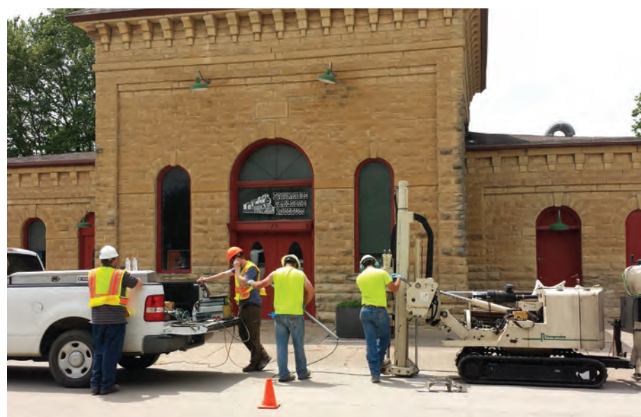
Members of GSI Engineering of Wichita, KS, and the Kansas Department of Health & Environment (KDHE) run an OIP-G log in front of the former Manufactured Gas Plant (MGP) building in Wellington, KS, which has been converted to a railroad museum.
