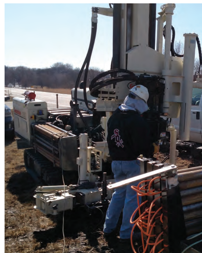
Bottom Right: Driller Doug Churchwell performs CPT research for pile design at a bridge over the Platte River using the Nebraska Department of Transportation’s new Geoprobe® 3230DT.
