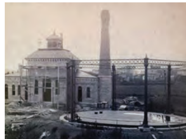
The Wellington, KS, Manufactured Gas Plant (MGP) under construction circa 1886. Note the gas holder in the right foreground. It was destroyed and back-filled after the plant closed.
