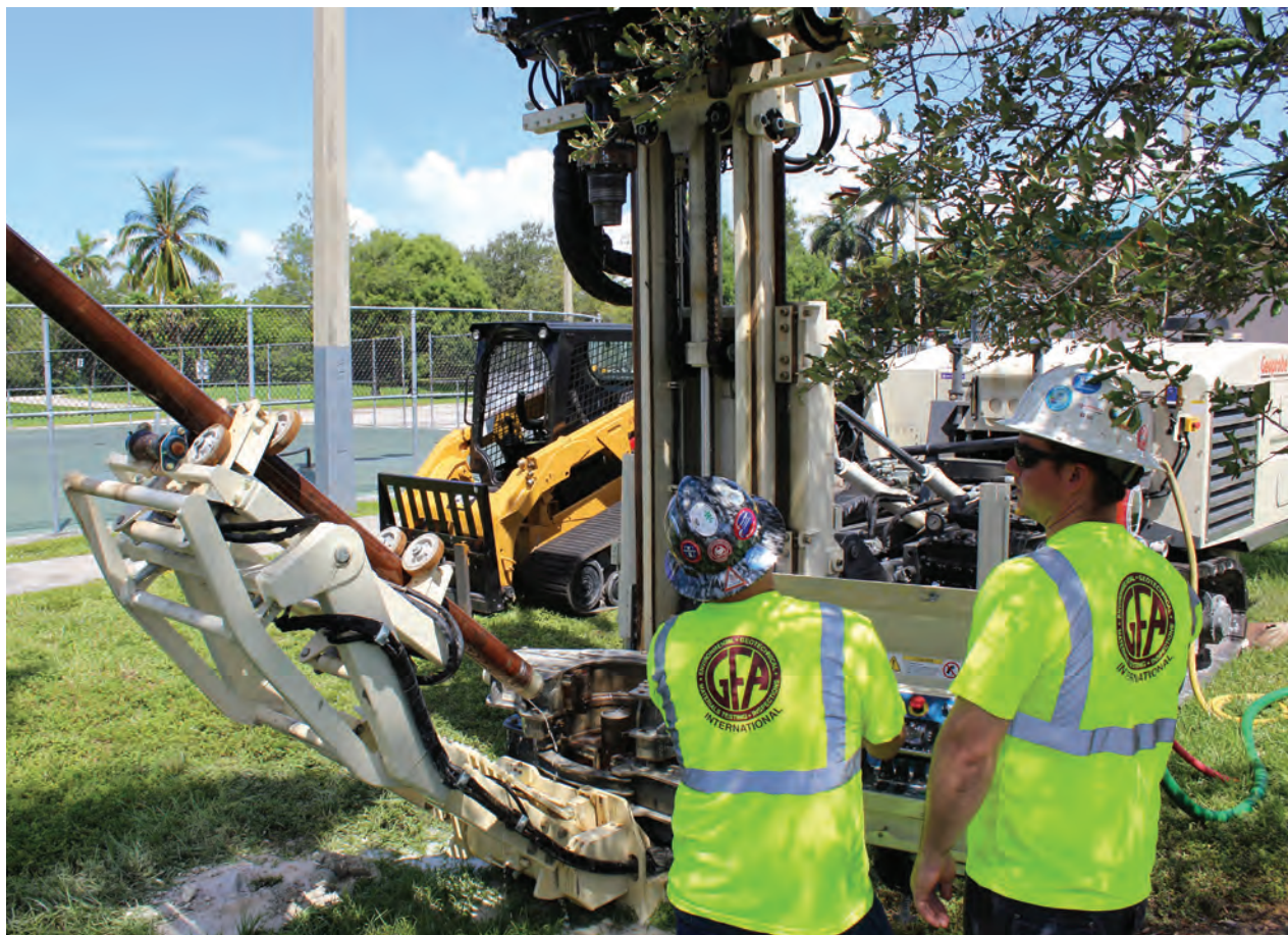
Lead Driller Brian McCord and Driller John Holdsworth use the 8150LS to install four deep salinity observation monitoring wells to a depth of 220 ft. in various locations throughout the City of Hollywood, FL. GFA International was retained by the City of Hollywood after using the 8150LS to complete a similar project in less than one week.
