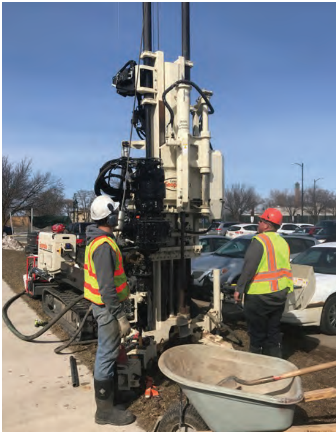
Shepler Well Drilling, Inc., completes split spoon sampling in Traverse City, MI, as part of a geotechnical site investigation for a new parking deck using their Geoprobe® 3230DT. The torque and pull back on the 3230DT put the crew at ease knowing they can retrieve their augers no matter what depth they reach on projects. Pictured are Operators Cole Shepler and Clint Bridson with Shepler Well Drilling.
