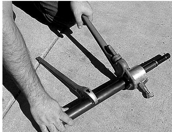
Figure 3. Tighten assembly with wrenches.
