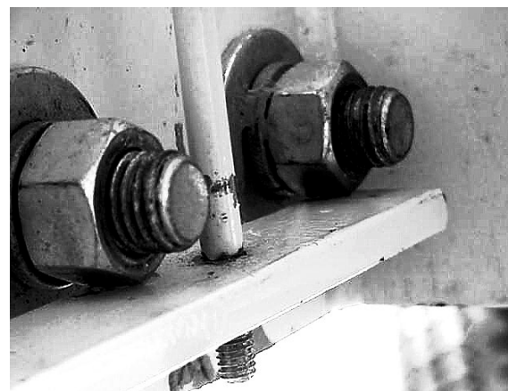
Figure 13. Holding brackets clamp to bolts on inside of 5410 foot.
