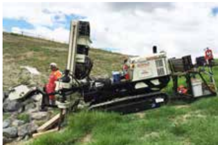
CPT compaction testing with the 6622CPT machine.
